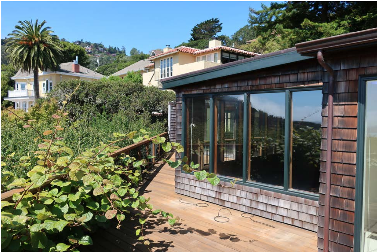
Fig.14 – 654 Sausalito Blvd. – Part rear from rear deck, looking northwest
