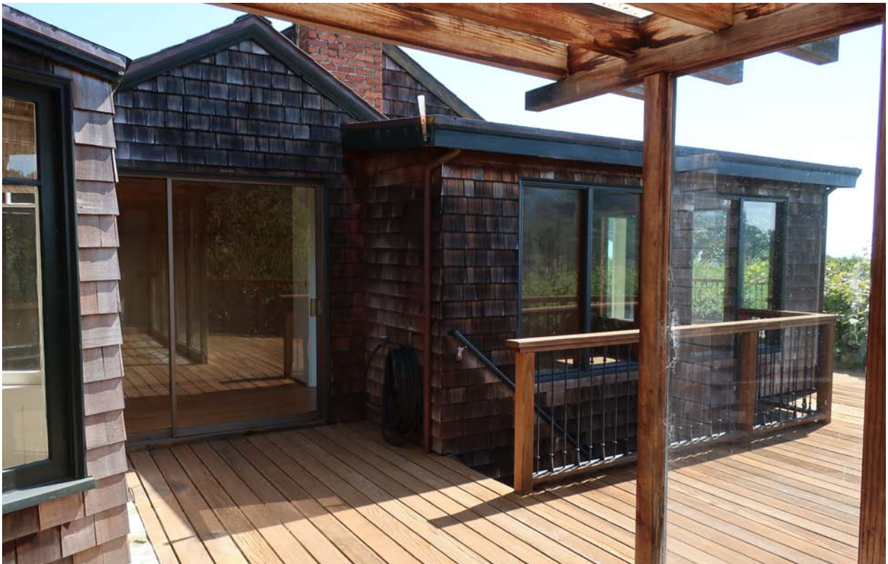
Fig.16 – 654 Sausalito Blvd. – West side from west side deck, looking east
