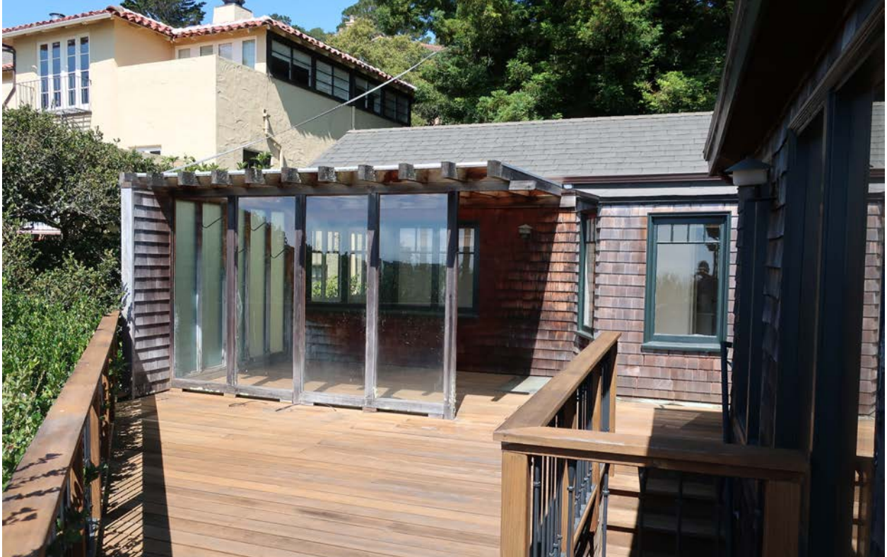
Fig.15 – 654 Sausalito Blvd. – Rear, west end, looking northwest
