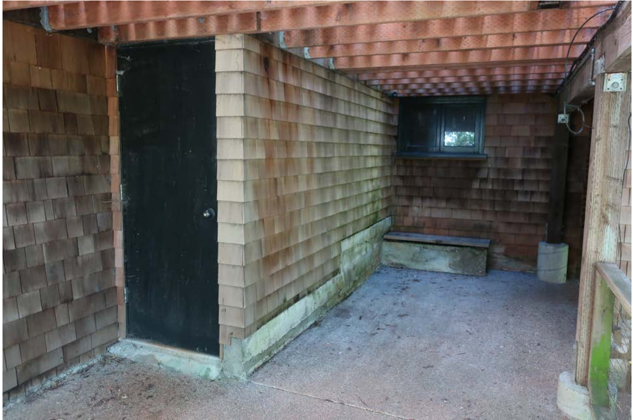
Fig.17 – 654 Sausalito Blvd. – West side, below deck, looking east
