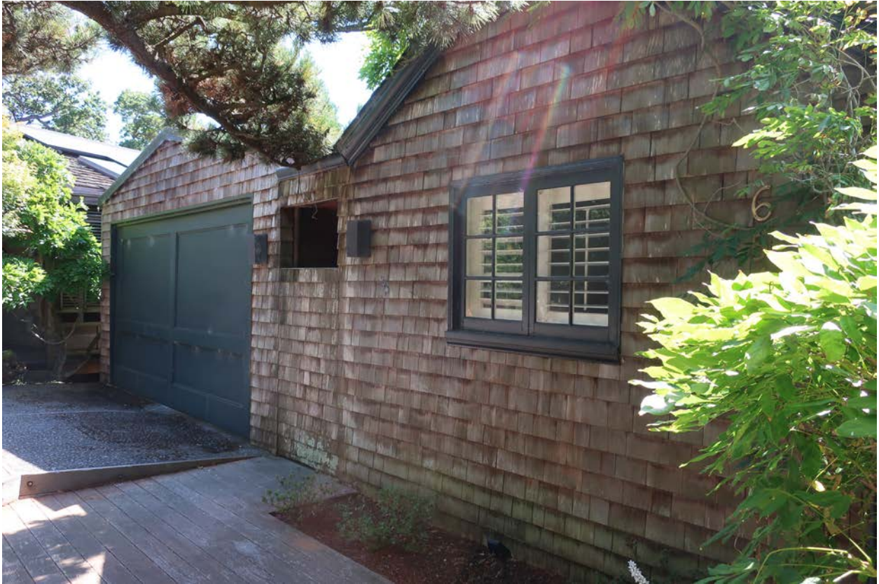
Fig.7 – 654 Sausalito Blvd. – Front, eastern part, looking east (MH, 2019, unless otherwise noted)
