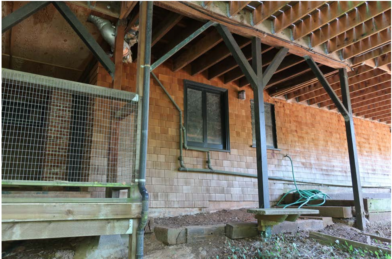
Fig.18 – 654 Sausalito Blvd. – Part rear from below deck, looking north
